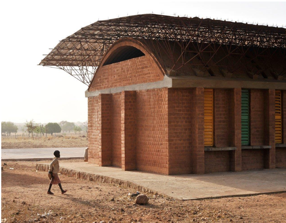
In 2001, Kéré erected the first school in his native village of Gando, Burkina Faso (West Africa). © Eric-Jan Ouwerkerk
